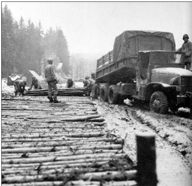
American engineers build a road in the Hurtgen Forest
